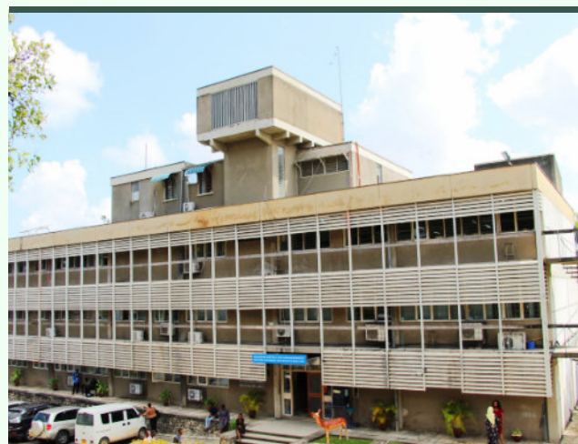
The building that hosted the Marine Biology Section, FAST and DASF. ©Rashidi Bilali
