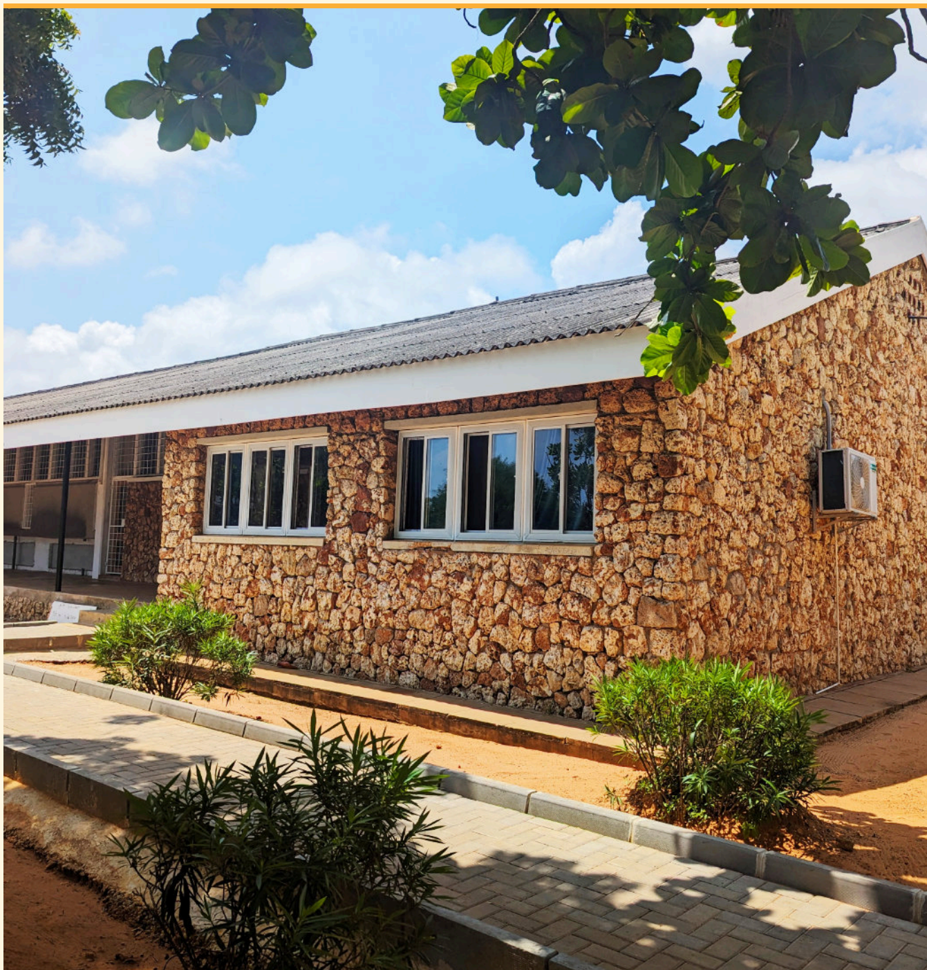
Laboratory building at Kunduchi Campus after rehabilitation. ©Rashidi Bilali
