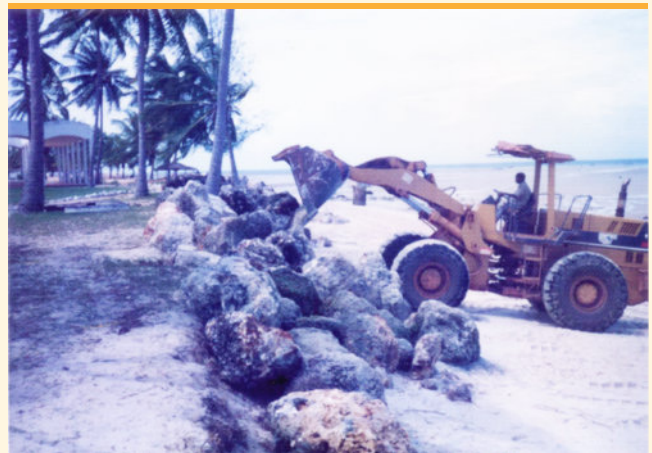
Land reclamation using stones at Kunduchi Beach Hotel in January 1996. ©Albogast T. Kamukuru
